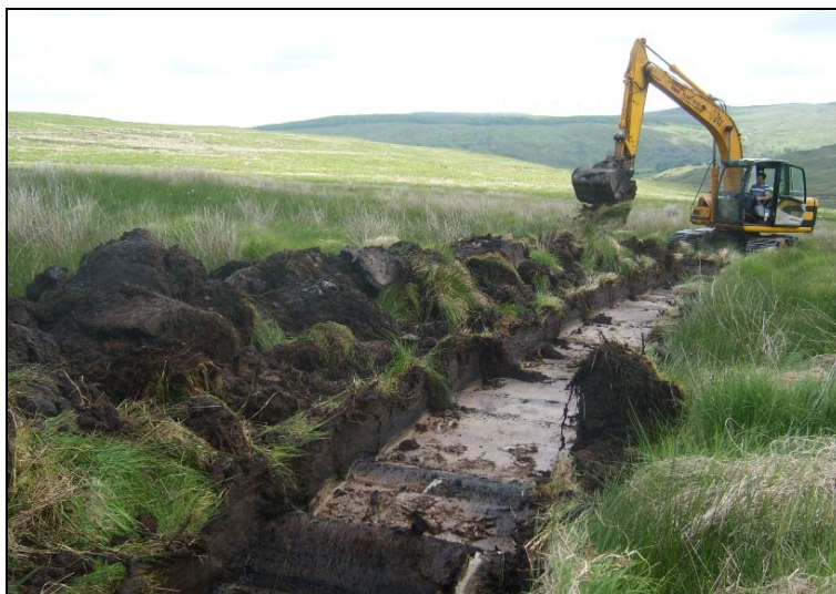
Plate 12: Test trenching at Turbine 6
