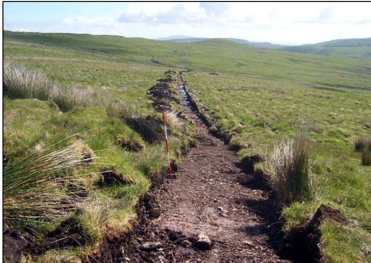
Plate 14: Test trench extending to Turbines 10 & 11
