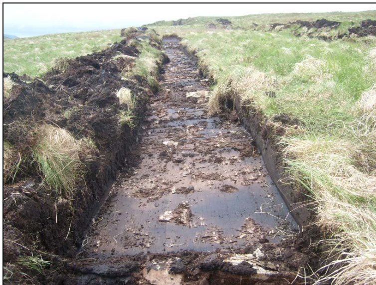
Plate 15: Test trenching at Turbine 10
