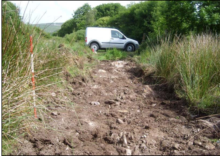
Plate 1: Trench in proposed temporary compound, view to north
