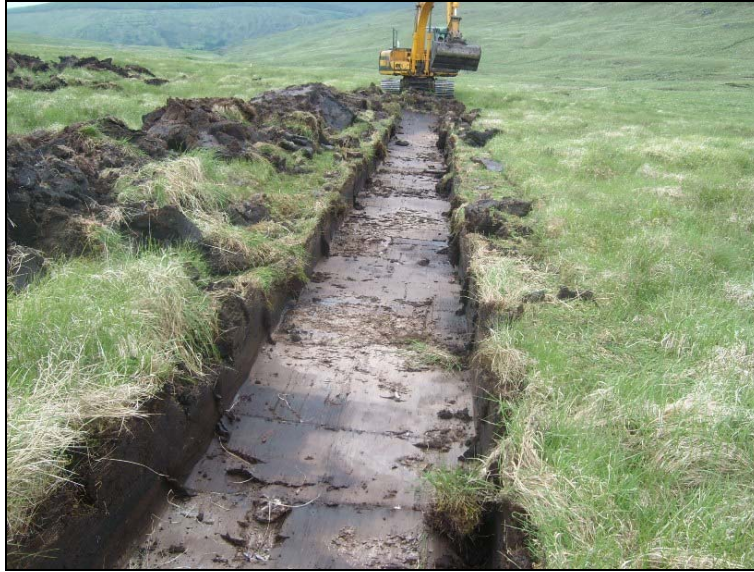
Plate 13: Test trenching at Turbine 8
