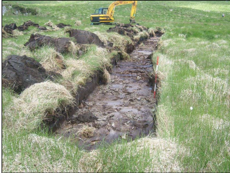
Plate 10: Test trenching at Turbine 3
